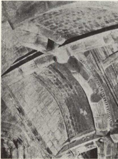
38. — HAGHBAT. Church of St. Nishan. Porch Vault.
