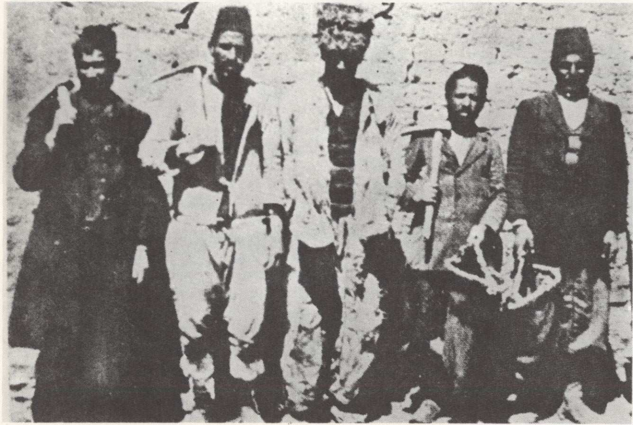
Tunnel digging group.
