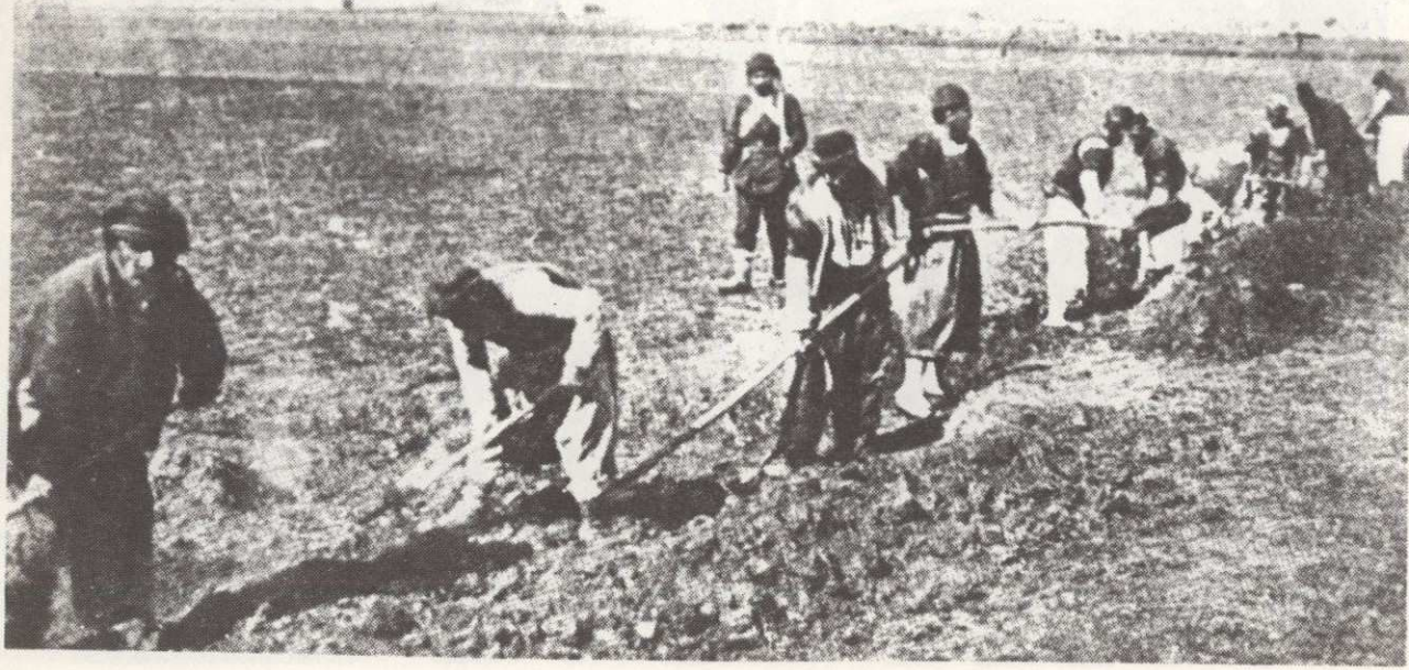
Preparing trenches for the fighters.
